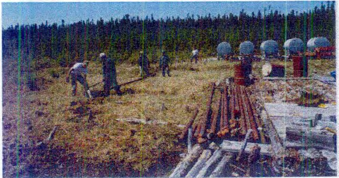
Site 221A Work crew dismantling 3 inch fuel pipeline.
