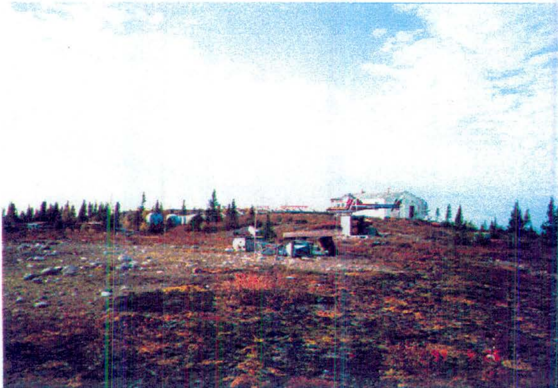
Site 330. View of crated radar parts and heaters. Operations building in background.
