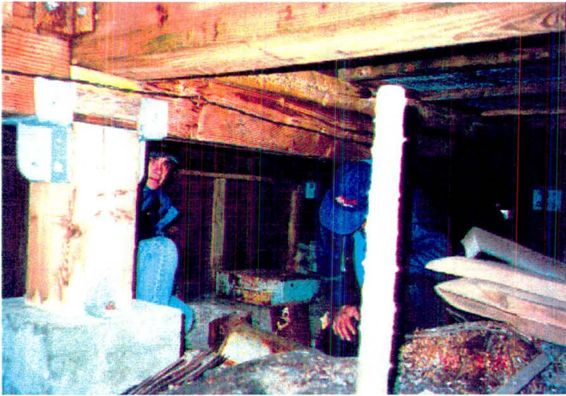
Site 333. Substructure of operations building and stored chemicals.
